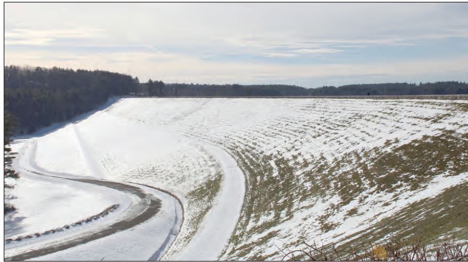
There are 40 caissons buried under this impoundment.
